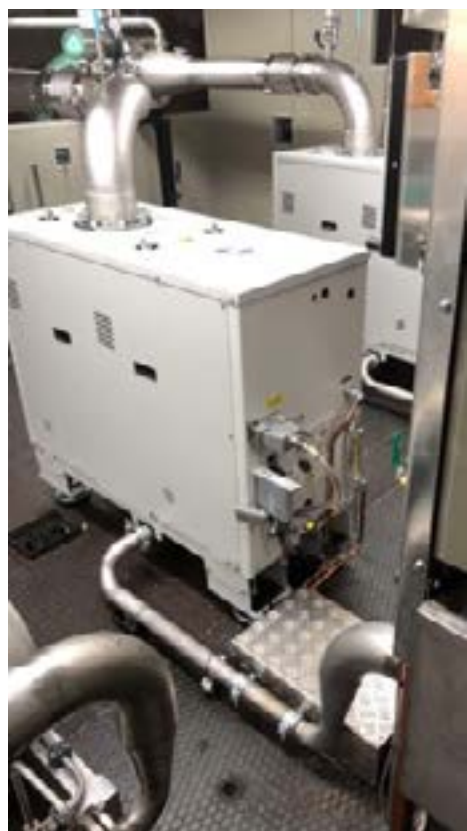
Multiple Edwards GXS450/2600 dry screw pump/booster combination installed at the Sandvik site on a sintering furnace.
