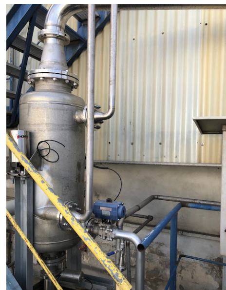
Inlet condenser to protect the EDC dry vacuum pump from any acidic liquid from jam production.
