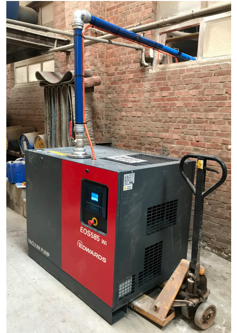
Edwards EOSi oil-injected screw vacuum pump
